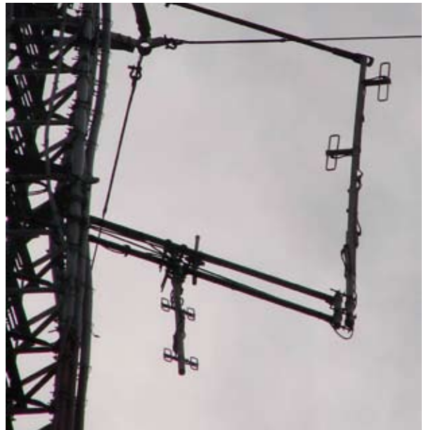
Here's the current setup on Moose Mtn. 2m on the right and 440 inverted.
